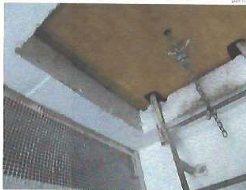
Reinforced Concrete Roof Deck
